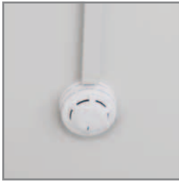
■ Explosion protected smoke detector
