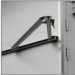
■ Door hold-open system with holding magnet
