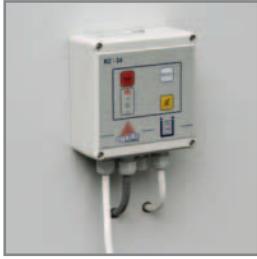
■ Electrical door hold-open system
